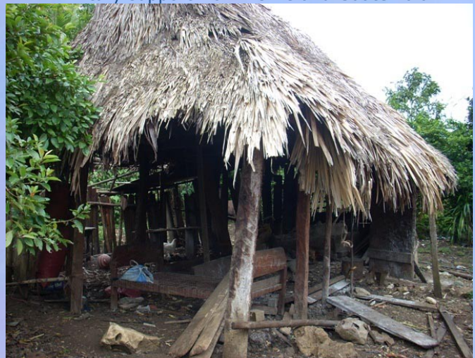
Dismantling of former house
