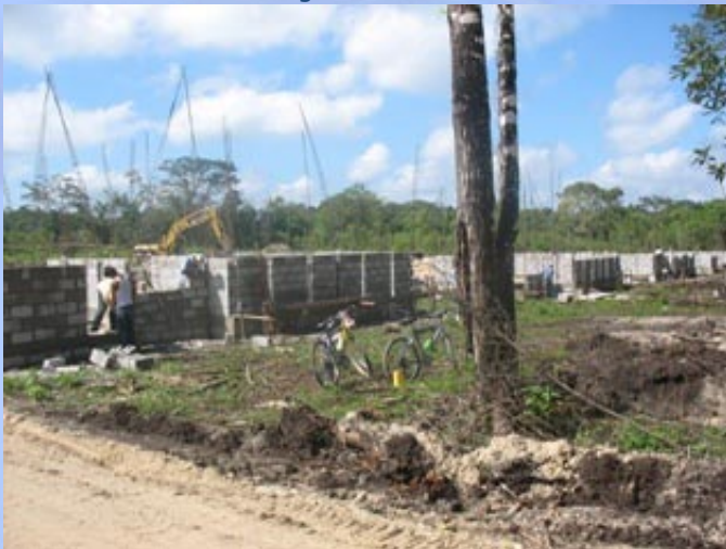
Rear view of construction
