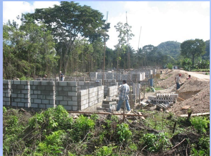
Front view of construction
