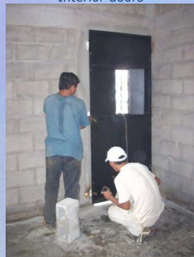
Installing entrance door
