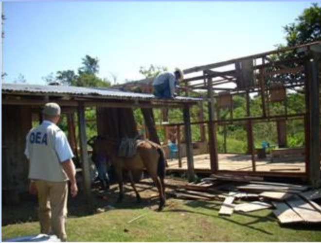
Dismantling of former house
