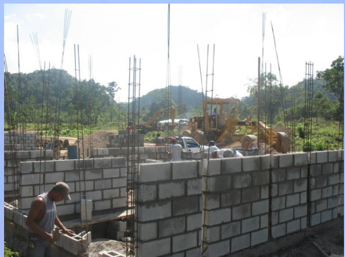
Construction of walls
